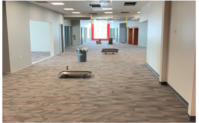
Carpet getting installed in the North classrooms 11/18/2022
