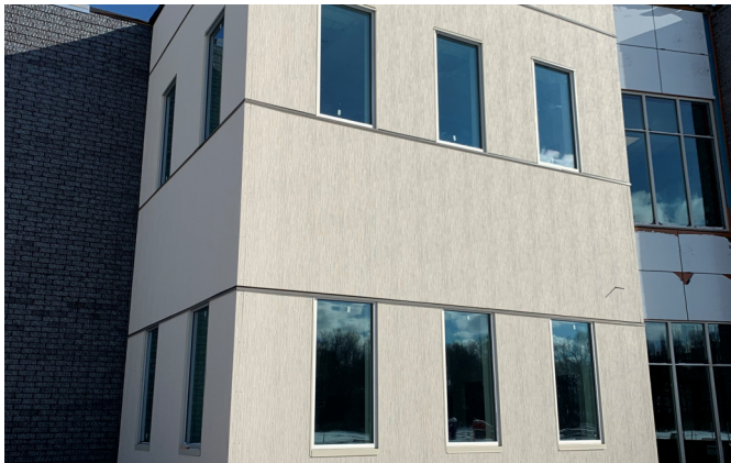
Completed siding on the North classroom wings 11/18/2022
