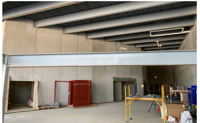
Main entrance lobby of the auditorium 11/18/2022
