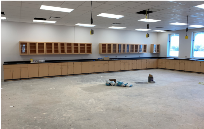
Science lab casework in the North classrooms 11/18/2022
