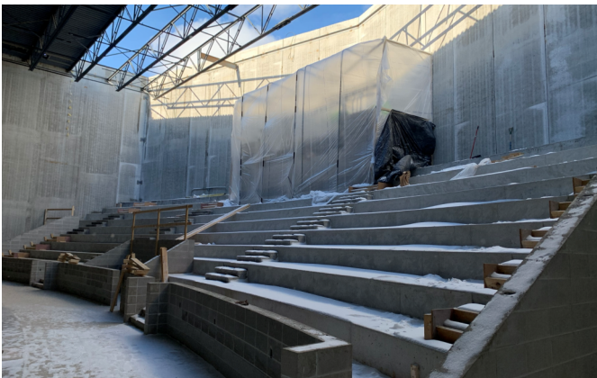
Masonry control room being built in the auditorium 11/18/2022
